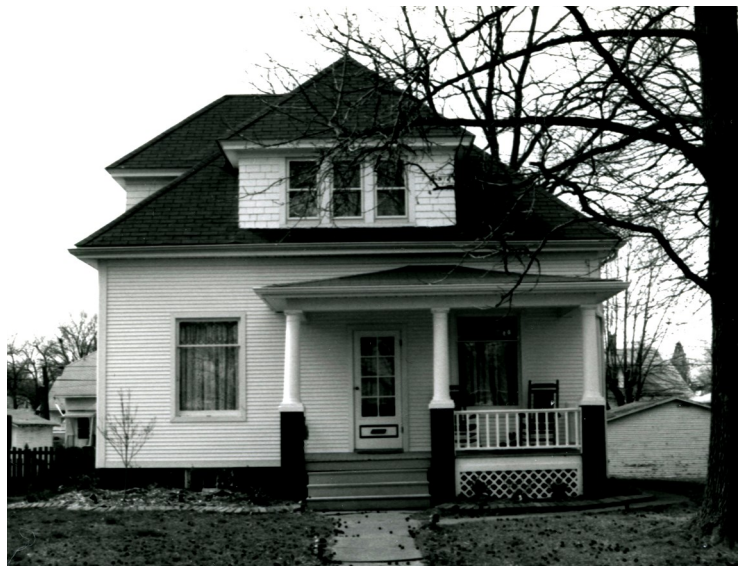
This photo of 1215 Emerson Avenue was taken in 1995 as part of a historic building survey conducted by the Edwardsville Historic Preservation Commission.
