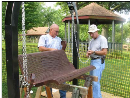
Gary Finke and Dennis Brown installing one of the new swings.
