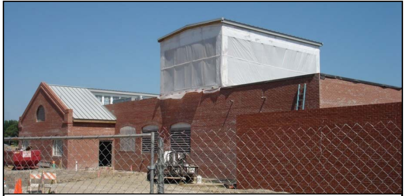
Progress on South Section of Jay Hoffman Center at Nelson
